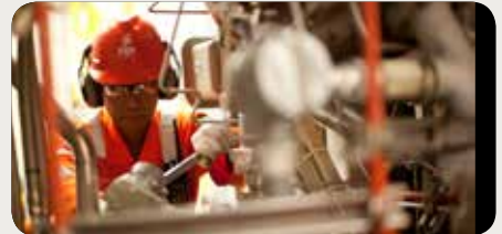
Gas infrastructure maintenance and operation operations by PGAS Solution.
