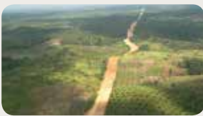
Transmission Pipeline Grissik-Pakardewa.
